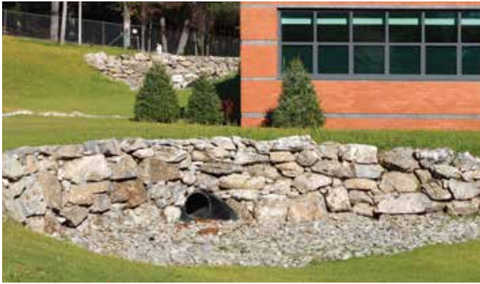
Stormwater swales vary in size and shape. They feature moss rock retaining walls and river round rock bottoms.
