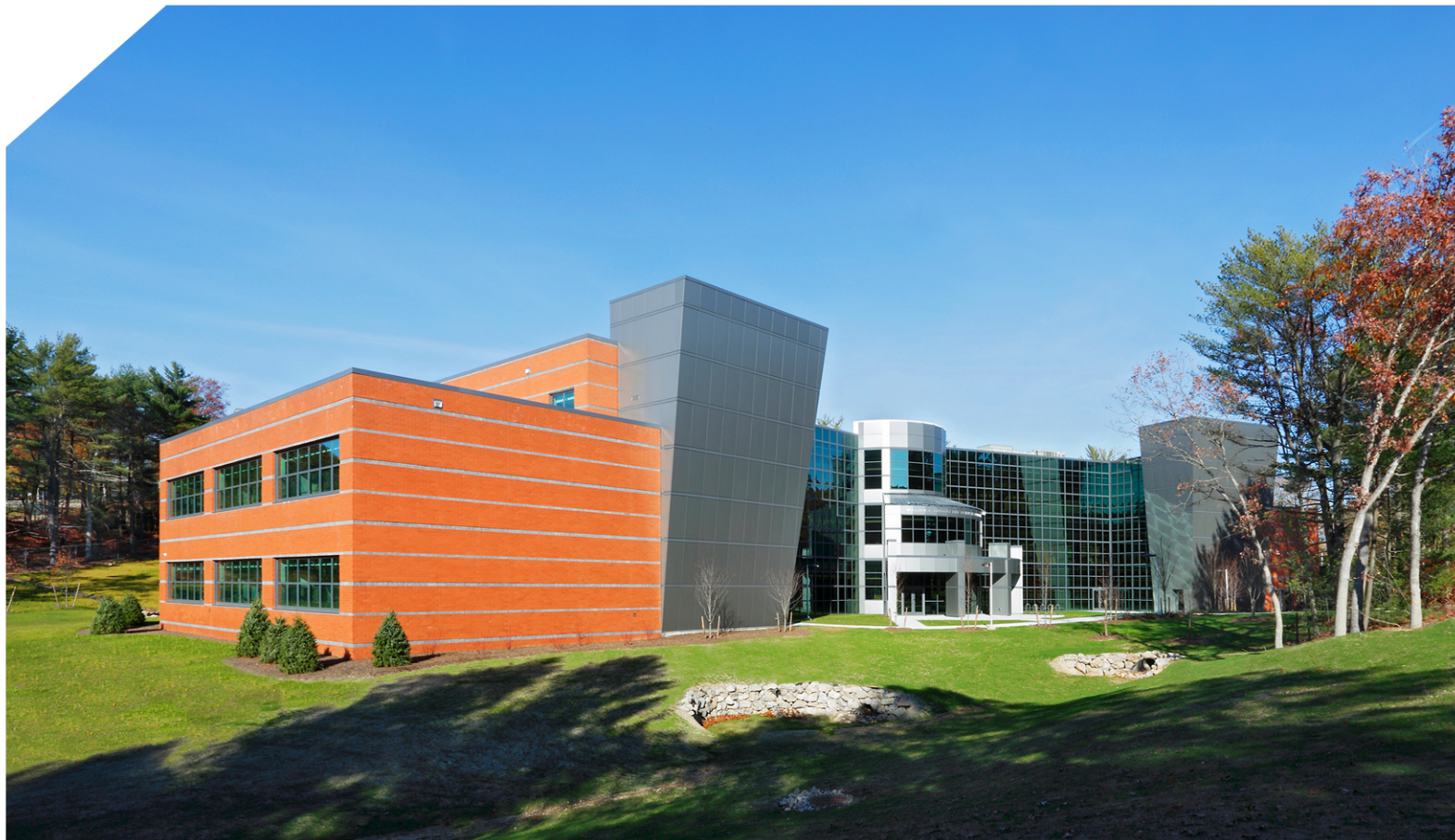
The Life Sciences Building features aluminum composite and glass curtain wall, and concrete masonry walls with a brick veneer. Photo: Tom Sibley/Wilk Marketing Communications
